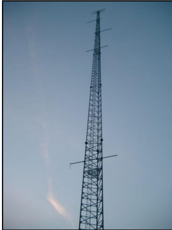
Figure 3-4: Example of a Meteorological Mast on a Wind Farm
