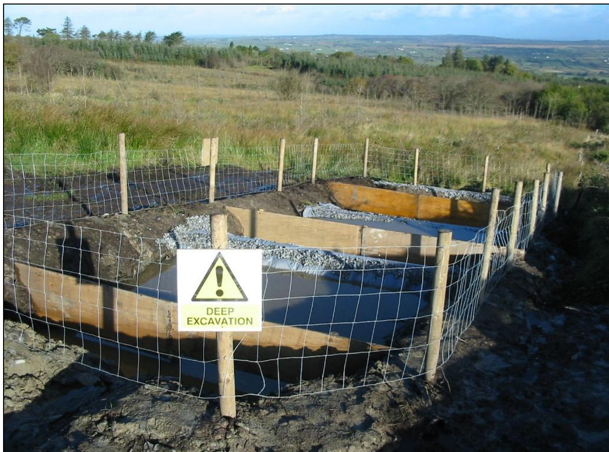
Figure 3-8: Typical Three-tiered Settlement Pond with Stone Filter
